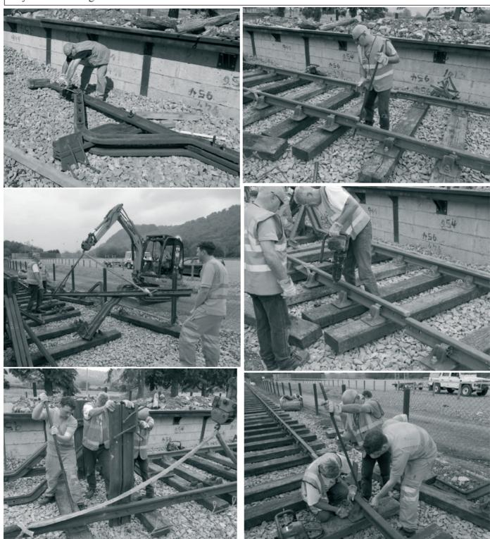
**Photos above:** (Top) Dave Trains tightens bolts on one side of the stop block (Centre) Here one side of the stop block is being lifted into position. (Bottom) Carwyn Rhys Jones, (left), Dave Lea and Dave Trains manhandle another part of the stop block into position
